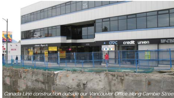
Canada Line construction outside our Vancouver Office along Cambie Street
